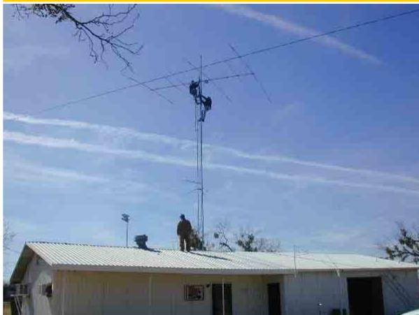
On February 2, several club members and Pecan Creek VFD helpers pulled down the old TH-5 yagi from the clubhouse tower and installed the 6-element TH-6. The boom on the TH-5 was not only bent, it was cracked and was held together only by the boom support cable.
